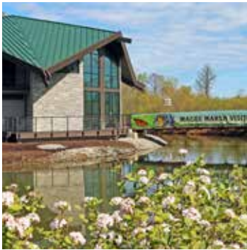
Magee Marsh Visitor Center, built in 1970 as the Sportsmen's Migratory Bird Center, was renovated in 2023.
